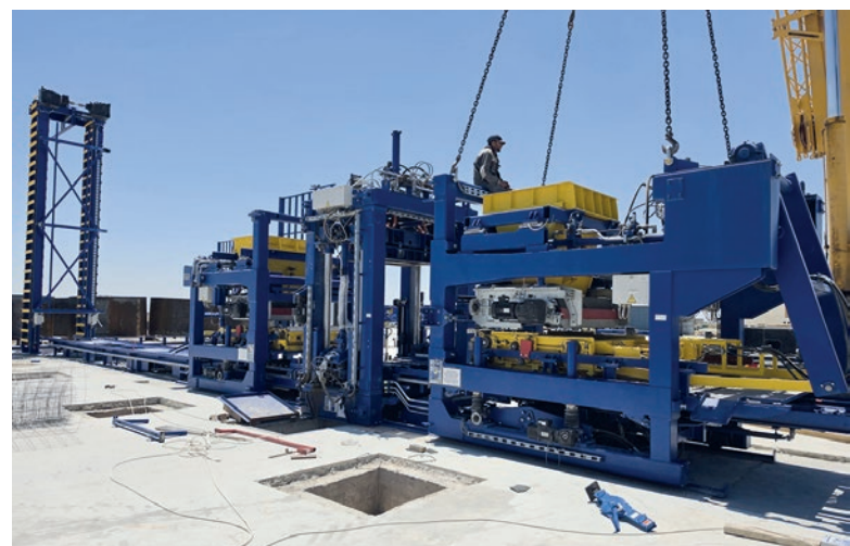
Arrival of the XL-R 9.1 in Algeria: the centrepiece of the plant is being installed.
