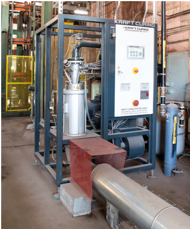
Kraft Vapor Generator 15-1S Replaces Old Boiler System
