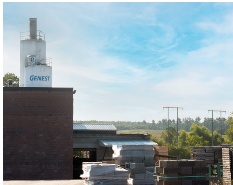
A View of the Yard at Genest in Beautiful Maine
