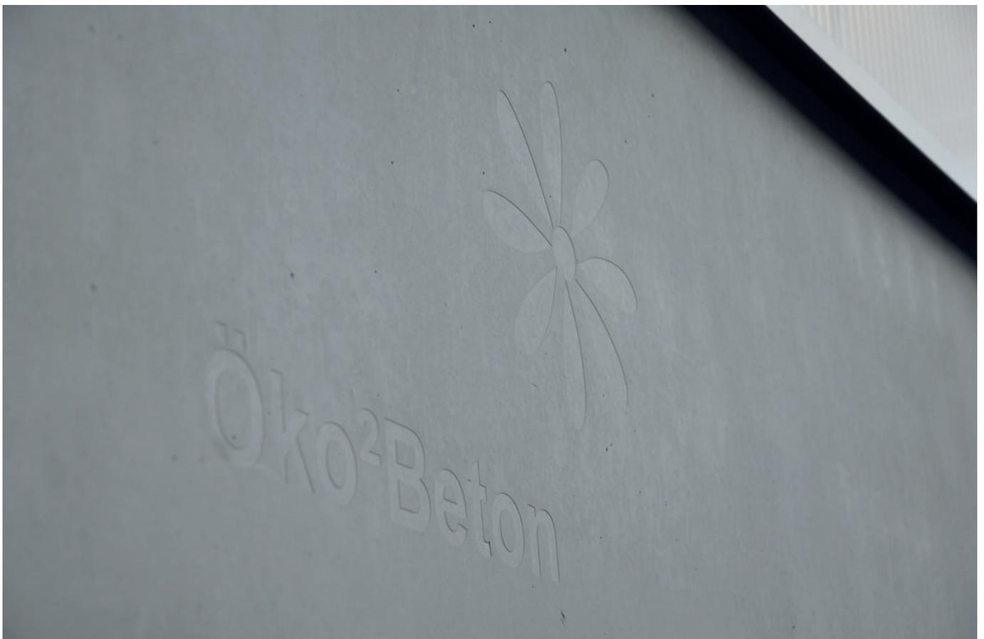
Fig. 6: Detail of an outer wall element made from eco-concrete in facing concrete quality
