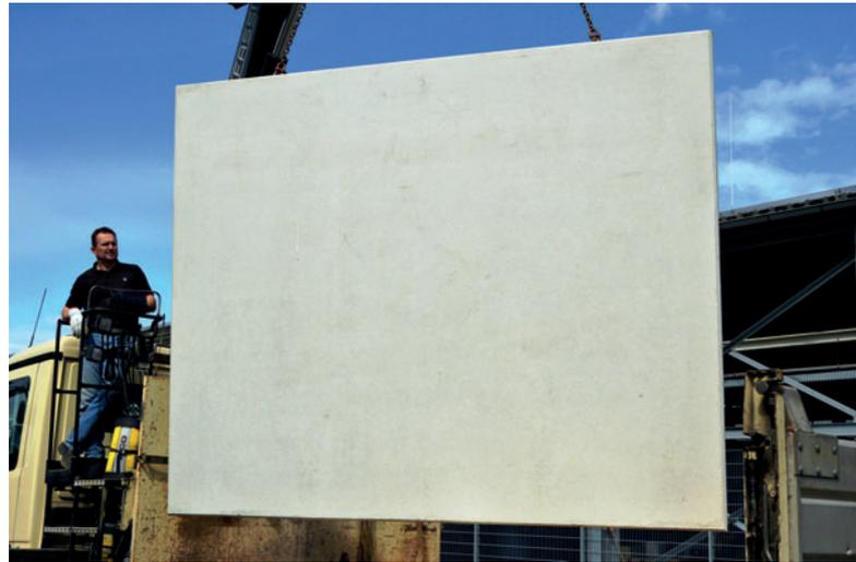
Fig. 5: Displacing an outer wall element made from eco-concrete
