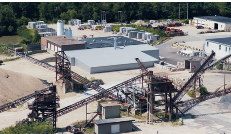
Genest Concrete Works installs the first patented Kraft Curing Rack System in the United States
