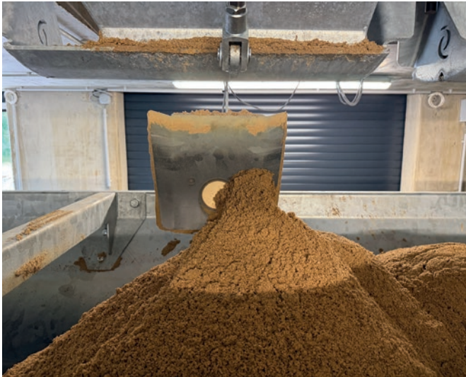
Moisture measuring probes are fitted to the dosing gates on the sand bins of the aggregate storage facility.
