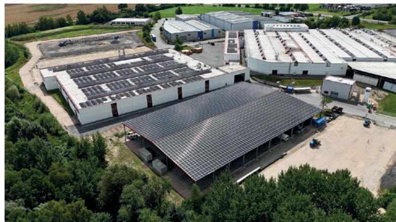
Kobra Carport – 180 covered parking spaces and 778 kWp of PV capacity
