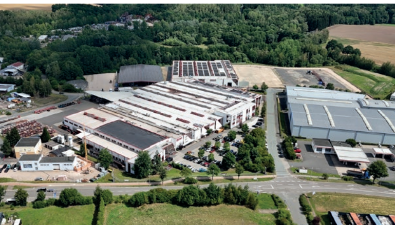
Kobra Formen GmbH – construction of two additional halls began in August 2026
