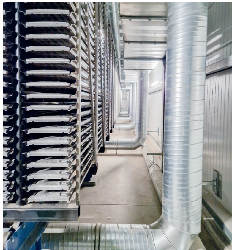
The controlled curing environment also contributes to more consistent hydration and strength development.
