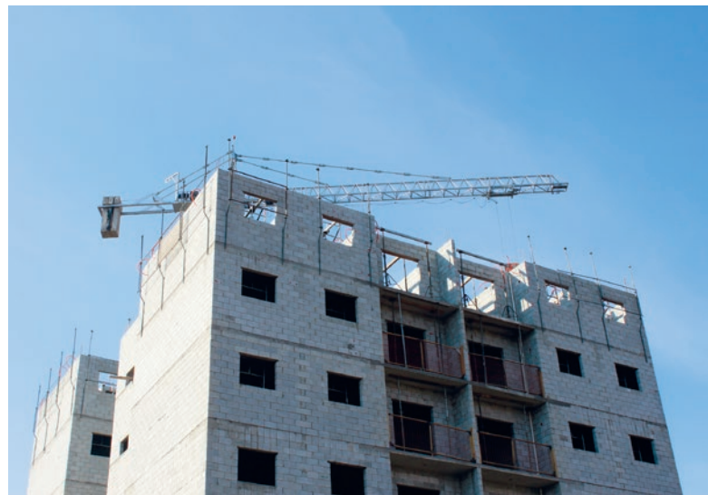
A building in which precast slabs with in-situ topping from the Brazilian pioneer have already been installed.
