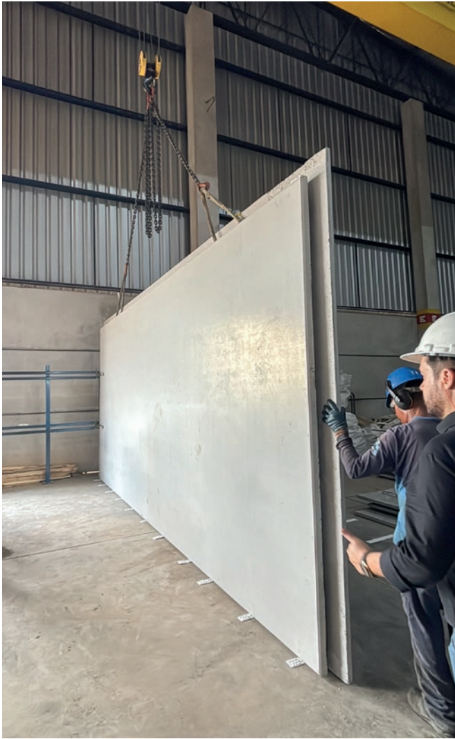
With the new turning device, the precast plant near São Paulo can now also produce double walls with a fair-faced concrete surface.
