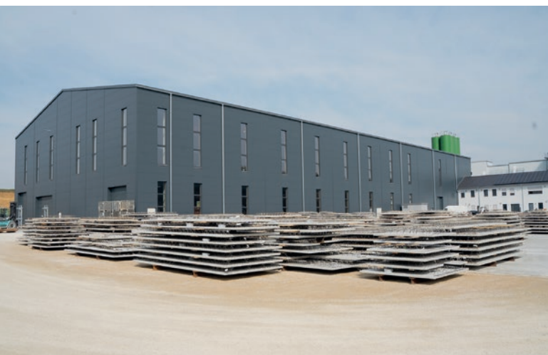
At Wöhrl's new production site, precast slabs with in-situ topping and double walls are manufactured using a modern pallet circulation system, with thermal and solid walls to follow.
