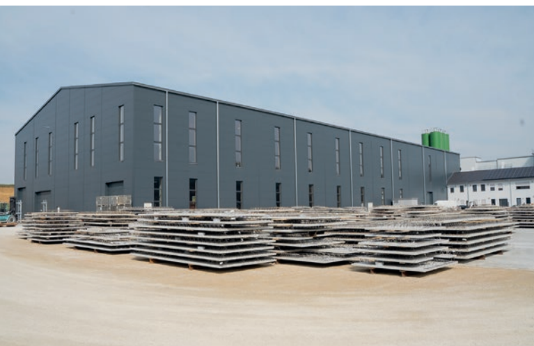
At Wöhrl's new production site, precast slabs with in-situ topping and double walls are manufactured using a modern pallet circulation system, with thermal and solid walls to follow.
