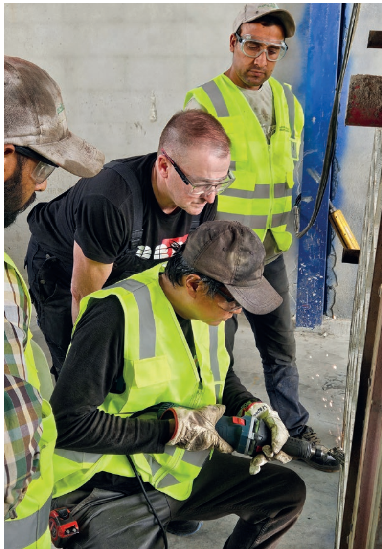
Grinding the lower edge of the mold after welding
