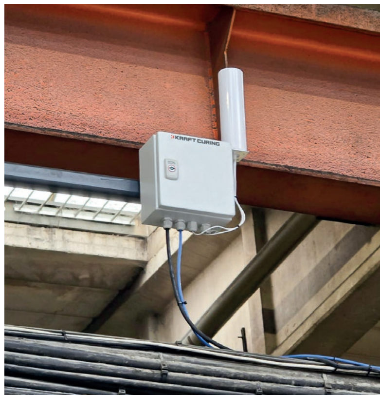
A wireless repeater placed throughout a factory or yard to ensure excellent signal strength throughout a large area.
