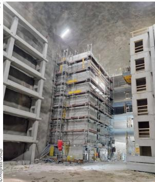
An extremely impressive infrastructure project is currently being realised beneath the streets of Merano: a six-storey underground car park in the Küchelberg tunnel. The 170 m long main cavern, which is fully accessible via a tunnel and offers direct pedestrian access to the city centre, is a technical masterpiece.
