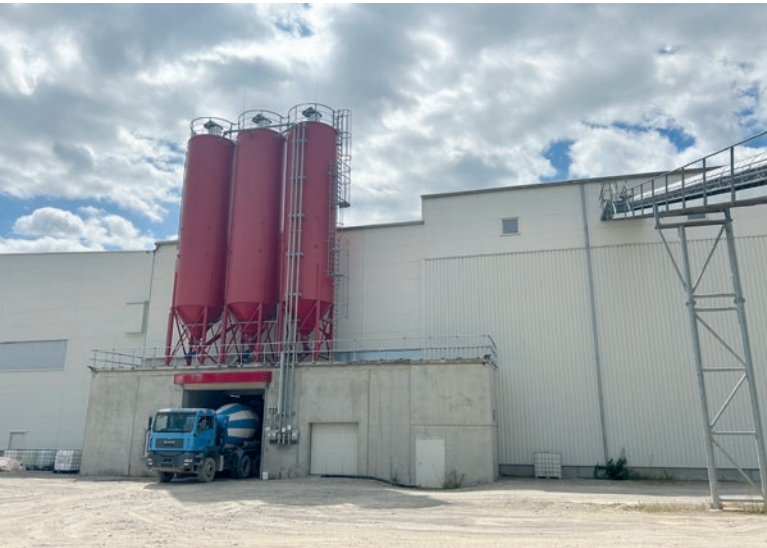
An additional part of the building serves as a foreman's office, storage room for admixtures and installation level for binding agent silos.
