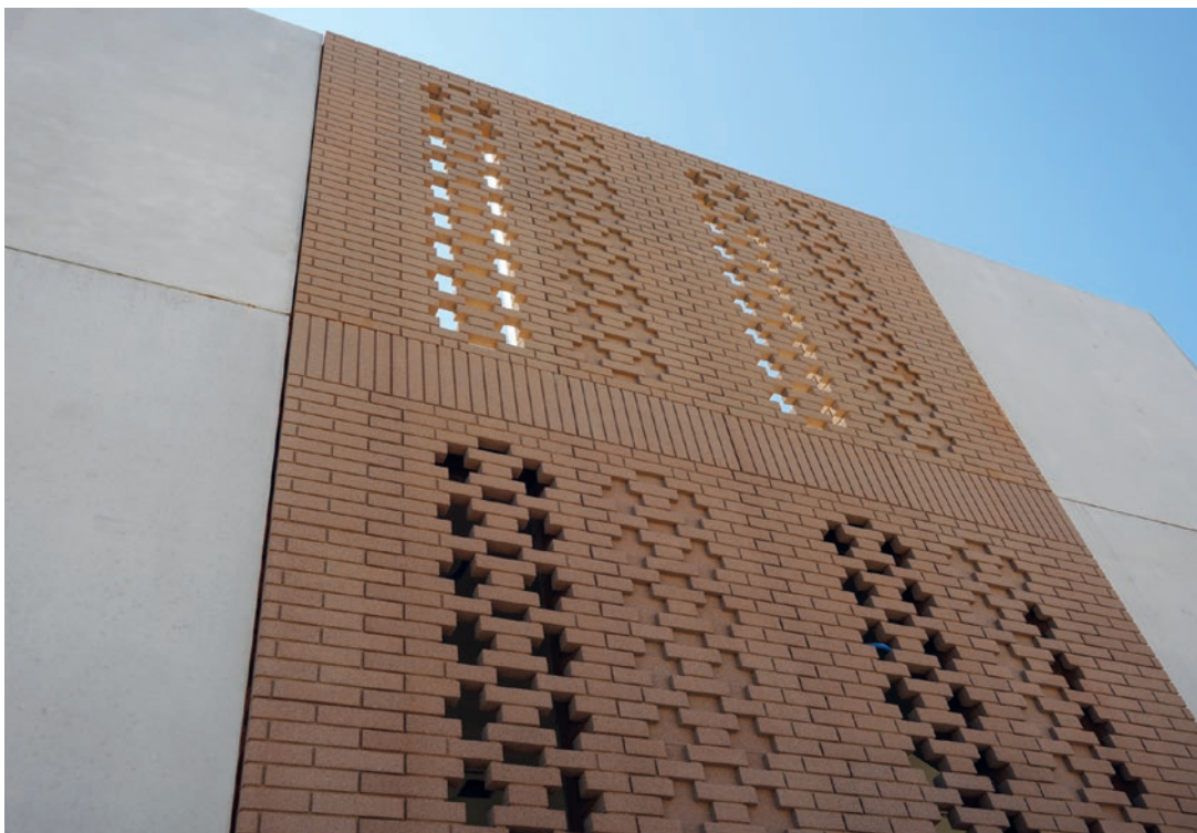
Façade element with 3D-printed brick texture.
