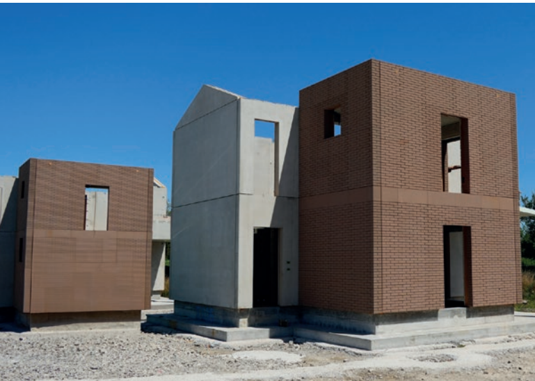
Unfinished holiday home with 3D-printed concrete façade elements.
