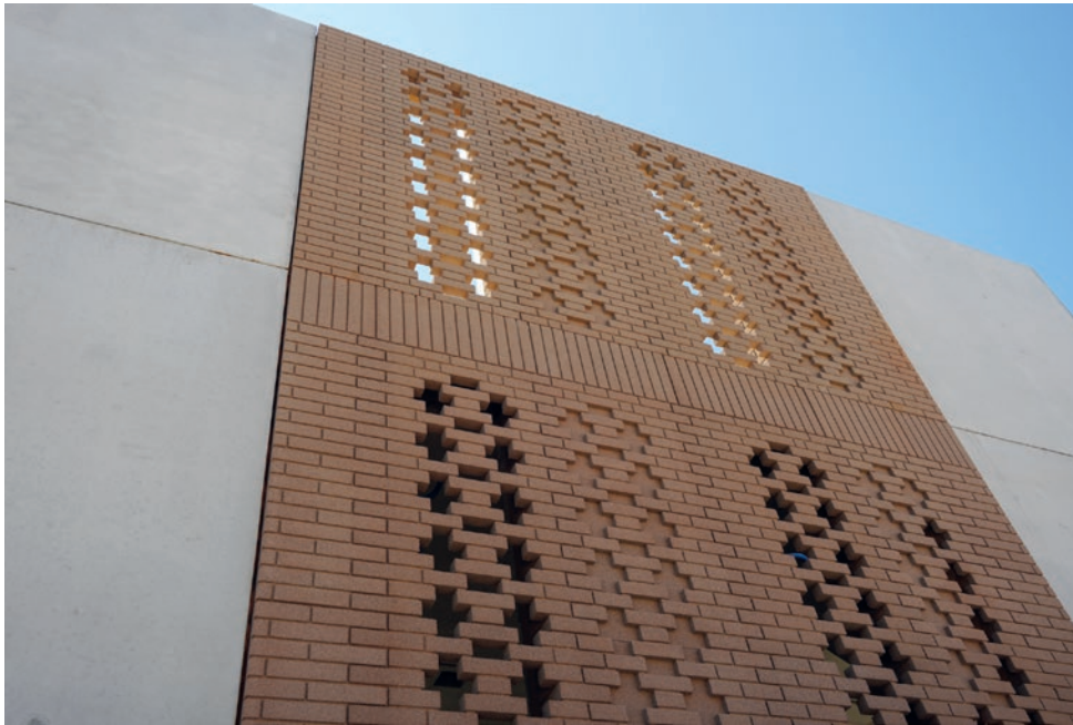
Façade element with 3D-printed brick texture.
