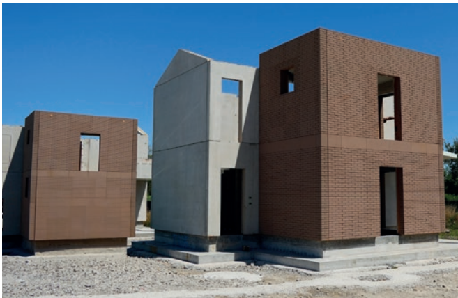
Unfinished holiday home with 3D-printed concrete façade elements.
