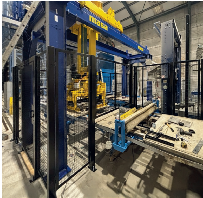
Installation of the new Masa Cuboter
