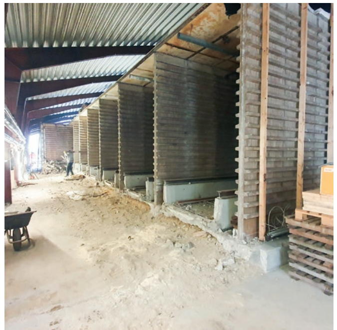
The chambers before the renovation in 2023
