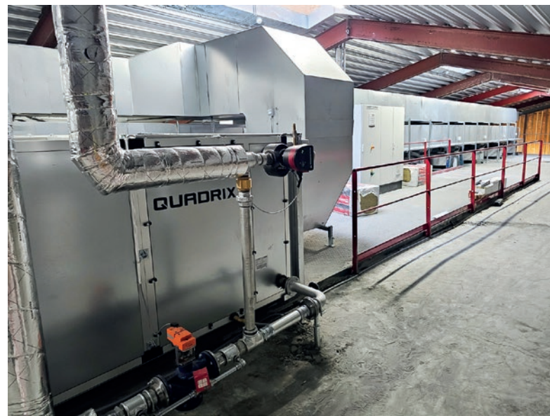
The Quadrix concrete curing system accelerates the curing process through the controlled addition of heat and moisture.
