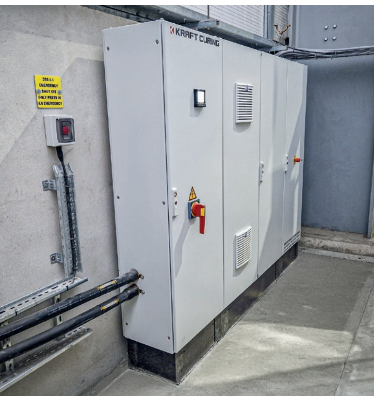
Left: KC 500 Convect-Air air heating and circulation unit connected to the original ducting. Right: Electrical load cabinet which provides multi-step control of the 500 kW electrical resistance heater, designed to provide a minimum curing temperature of 40 degrees Celsius year-round.
