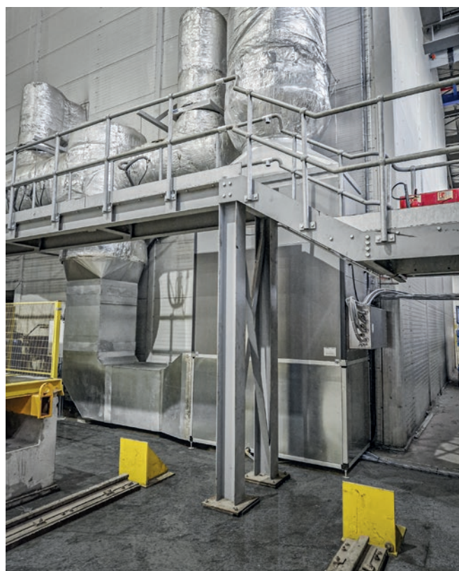
Left: KC 500 Convect-Air air heating and circulation unit connected to the original ducting. Right: Electrical load cabinet which provides multi-step control of the 500 kW electrical resistance heater, designed to provide a minimum curing temperature of 40 degrees Celsius year-round.
