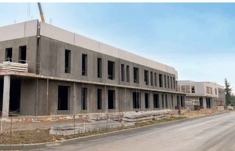
Installation of wood-concrete walls, double walls with low CO 2 content and Isopré walls at the Bouygues hospital in Tours
