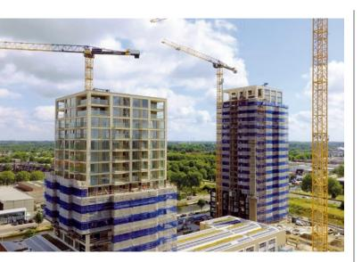
High-quality precast concrete elements from Lammers Beton in use at the De Caai project in Eindhoven combining modern design and efficient construction.
