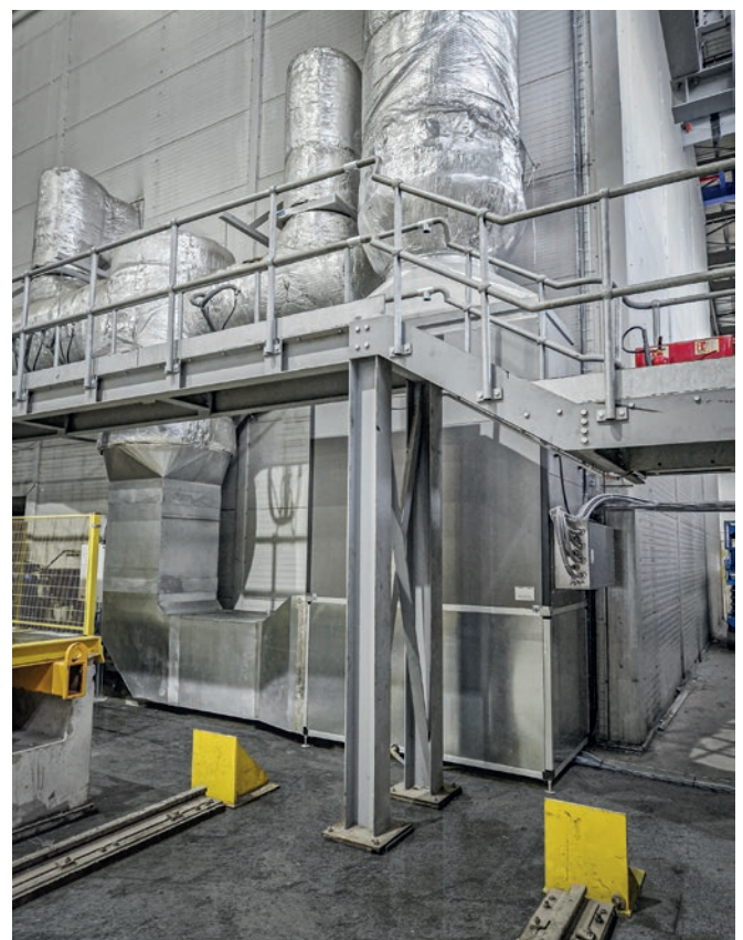
Left: KC 500 Convect-Air air heating and circulation unit connected to the original ducting. Right: Electrical load cabinet which provides multi-step control of the 500 kW electrical resistance heater, designed to provide a minimum curing temperature of 40 degrees Celsius year-round.
