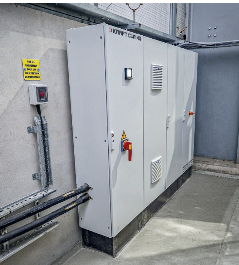
Left: KC 500 Convect-Air air heating and circulation unit connected to the original ducting. Right: Electrical load cabinet which provides multi-step control of the 500 kW electrical resistance heater, designed to provide a minimum curing temperature of 40 degrees Celsius year-round.
