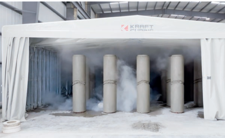
A retractable enclosure with integrated vapor curing in action.
