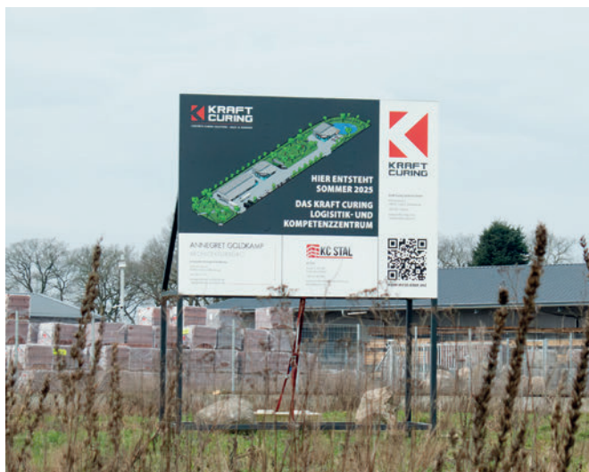
Site of the future expansion of the Kraft Curing Headquarters.
