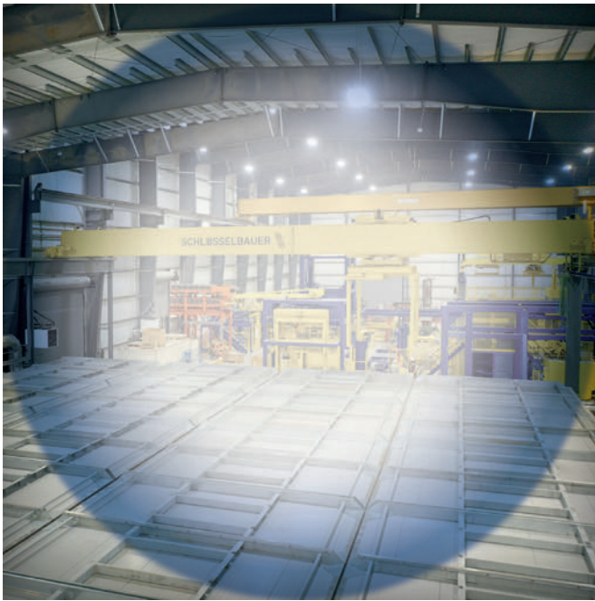
Curing chambers with automatic filling
