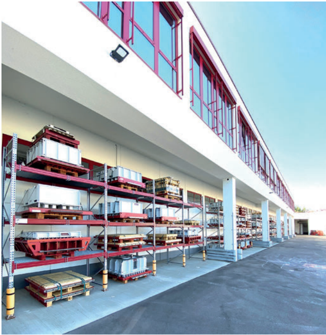
Dispatch warehouse with new moulds
