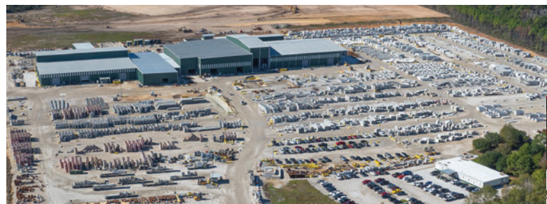
The AmeriTex site in Houston - the home of the new Magic manhole riser production system
