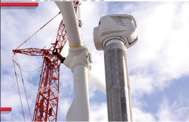
100 METER TALL (328 FEET) PRECAST WIND TURBINE TOWER
