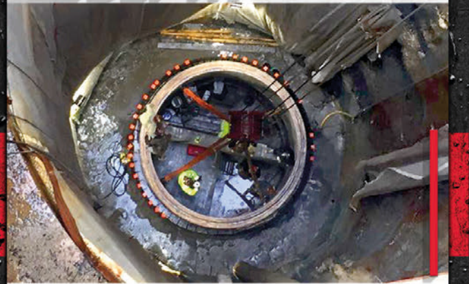
160 FEET DEEP (48.8 METER) UTILITY ACCESS 14 FEET (4.3 METER) DIAMETER PRECAST MANHOLE
