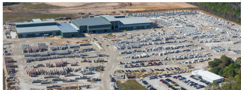
The AmeriTex site in Houston - the home of the new Magic manhole riser production system
