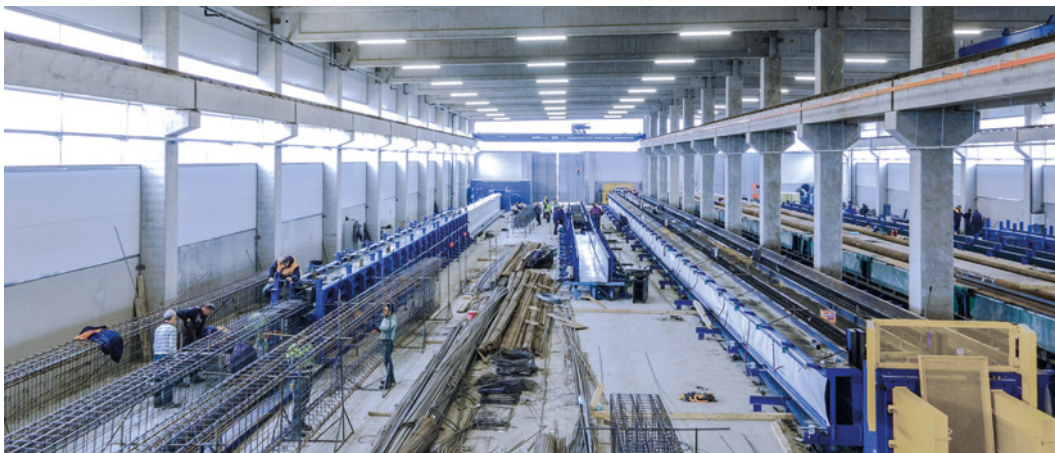
The various moulds installed are between 32 and 62 meters long.
