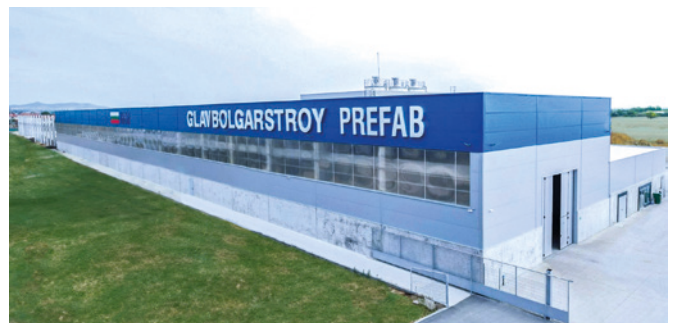
Glavbolgarstroy Prefab is part of Glavbolgarstroy Holding, a leading Bulgarian construction company and represents one of the most advanced precast plants in the country.
