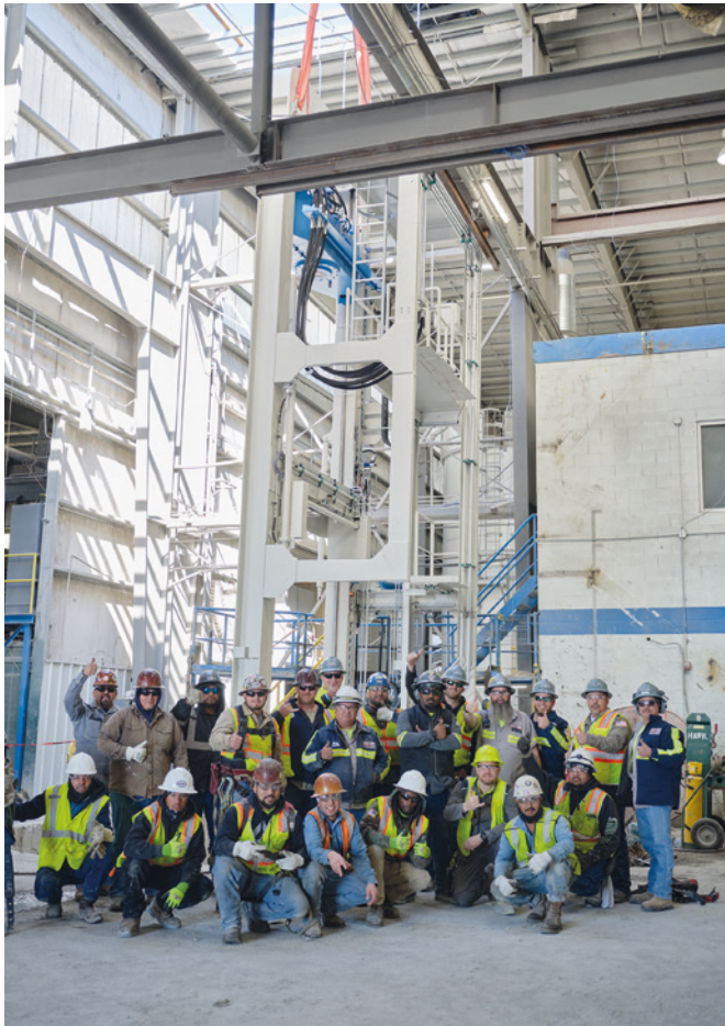
Successful Radial Press Replacement
