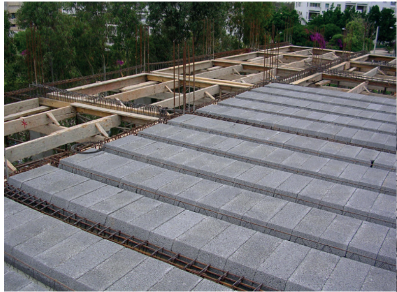
Installation situation floor blocks on site
