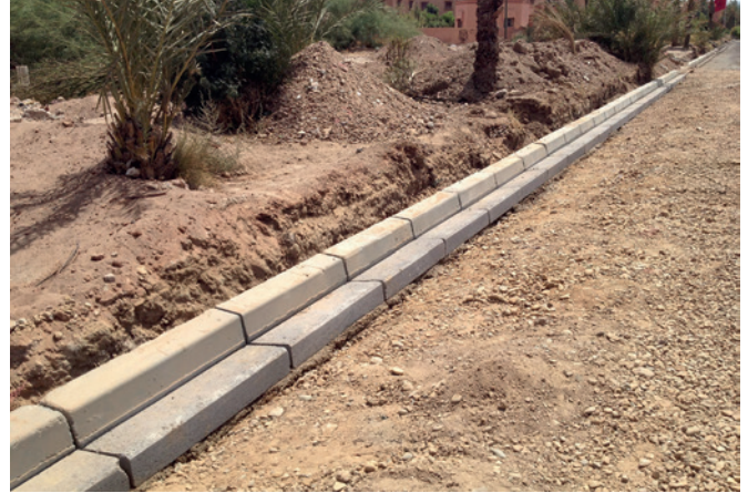
Construction site near Marrakech
