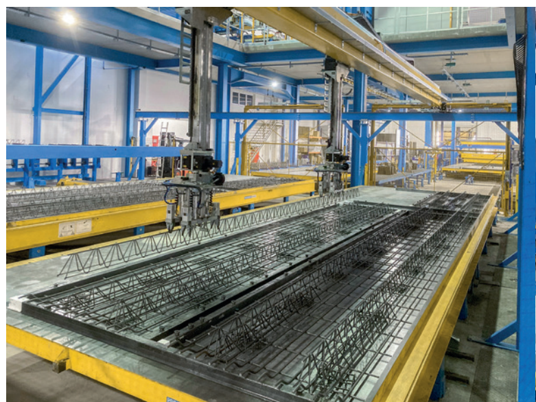
With flexible logistics solutions such as the laying robot, the reinforcement can now be transported and laid without heavy physical labour.
