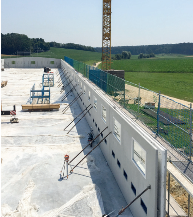
Thermal walls are also used in agricultural construction, as here for a poultry house.
