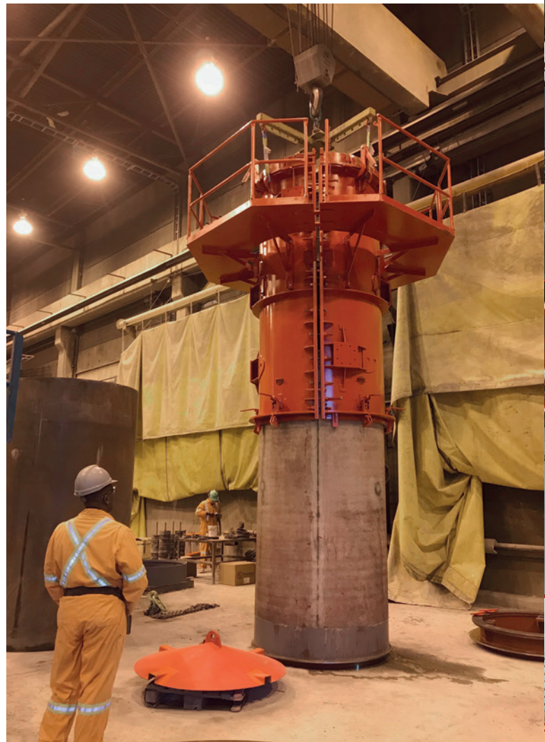
Demolding of the mold jacket - Cured Jacking pipe on base pallet
