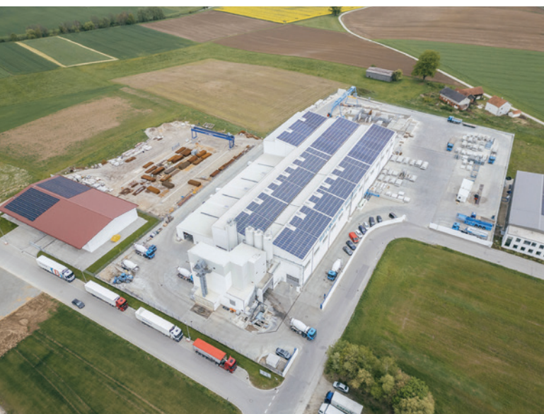
The Rembeck concrete plant, which was newly built in 2012, has now been made fit for the future with a completely new circulation plant from Progress Group.
