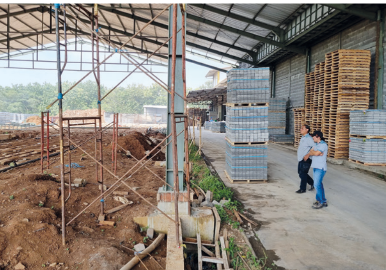
Foundation work for the new concrete block and paver line. On the right is the hall of the Hess RH 1500-3 concrete block and paver machine, purchased in 2010.
