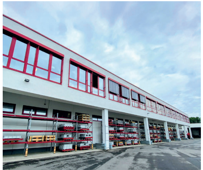
The dispatch rack of the Kobra company in Lengenfeld
