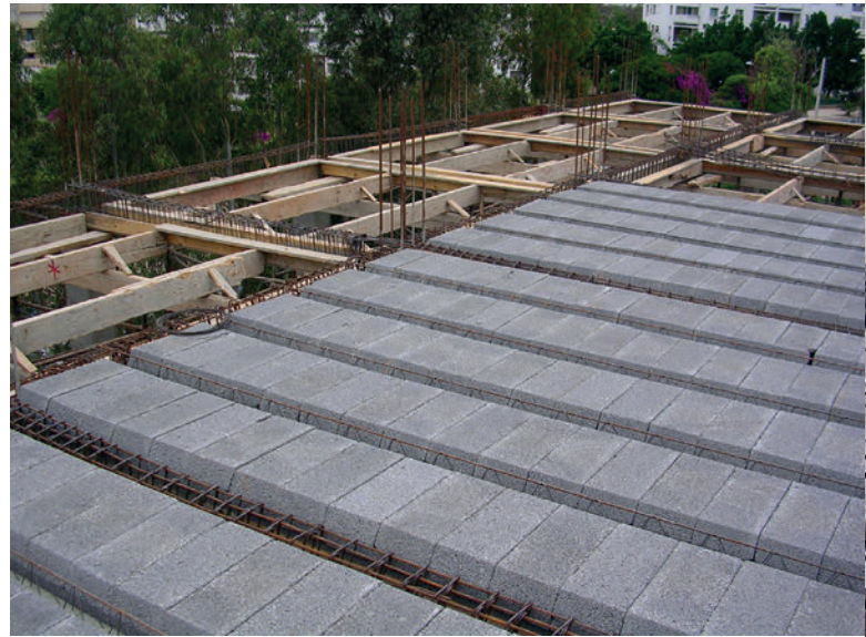
Installation situation floor blocks on site
