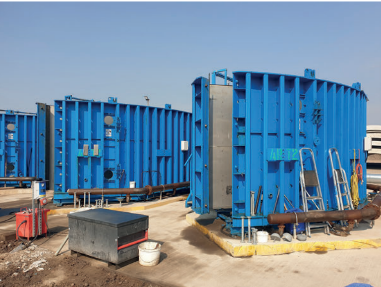
Outdoor temporary casting area allowed the customer to meet the project delivery schedule while awaiting completion of the permanent cast facility.
