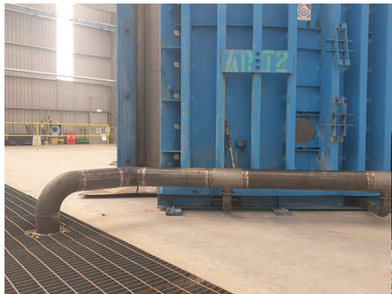
Primary Curing in the Permanent Facility - Pipe trenches keep the production floor free from obstructions. The vapor is always delivered at ground level, directly under the form for best temperature consistency.
