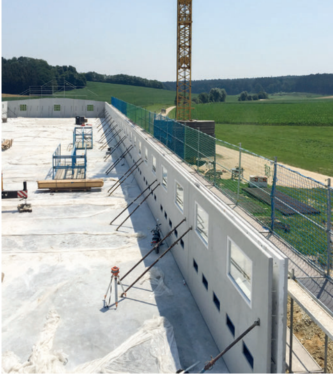
Thermal walls are also used in agricultural construction, as here for a poultry house.
