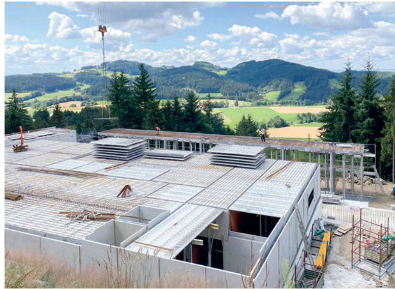
The mountain inn in the Edelwies leisure park in the Bavarian Forest is currently being built with the precast elements from the new factory.
