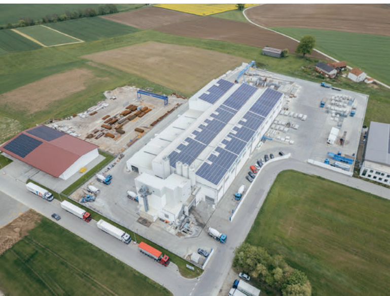
The Rembeck concrete plant, which was newly built in 2012, has now been made fit for the future with a completely new circulation plant from Progress Group.
