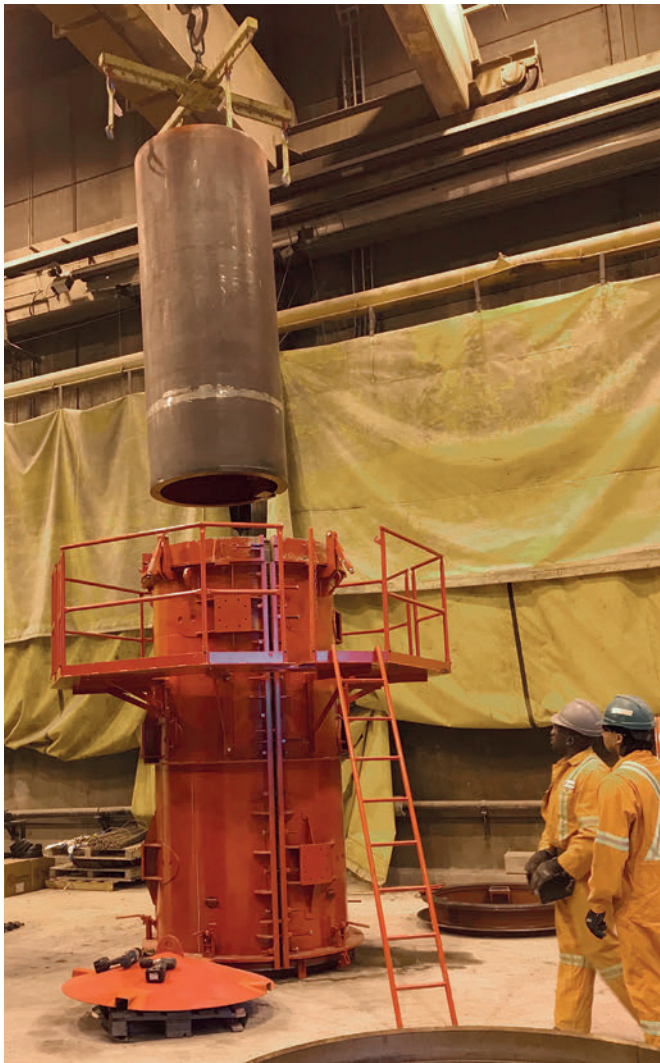
Demolding process begins - Removal of the mold core
