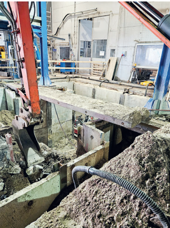
Foundation preparation (Hardenberg)
