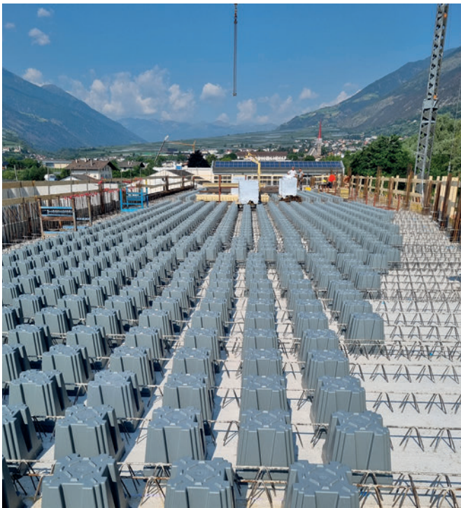
The Green Code Eco Slab® is completed on the building site with the GC top, i.e. the upper half of the recess body, which is available in different versions for different slab thicknesses.
