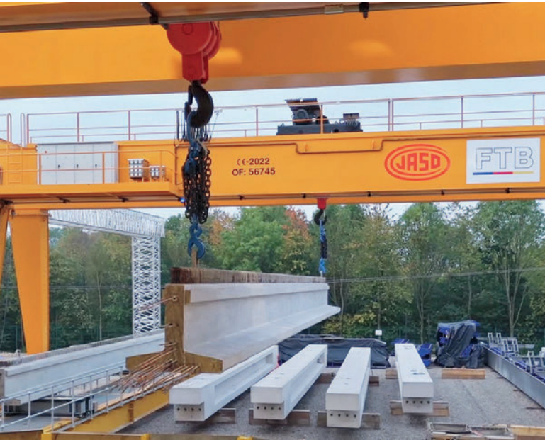
The facility uses a total of four benches to produce up to ten bridge beams each day.
