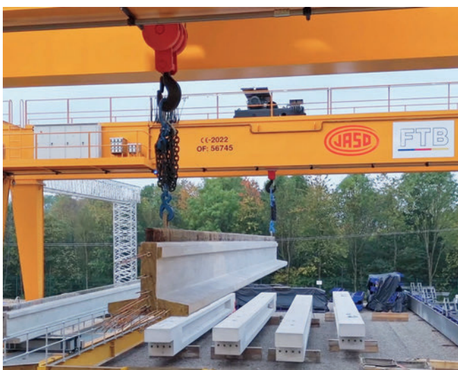
The facility uses a total of four benches to produce up to ten bridge beams each day.
