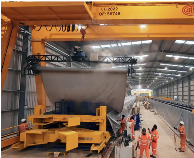
The motorized tarp roller moves along the form by way of the overhead crane, evenly unrolling the curing tarp.
