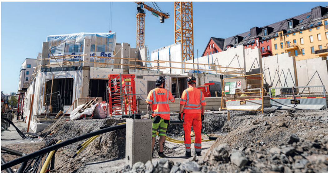
This residential project Persikan in Södermalm is currently being built with precast elements from the new factory in Hallstahammar.
