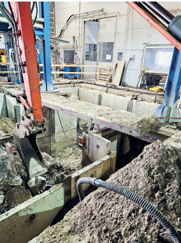
Foundation preparation (Hardenberg)
