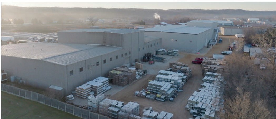
Rochester Concrete Products' new manufacturing plant at their Interlock Concrete location in Jordan MN
