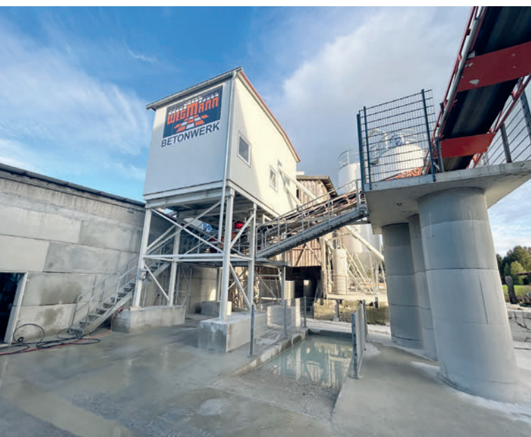
View of the new concrete mixing plant at Wegmann
