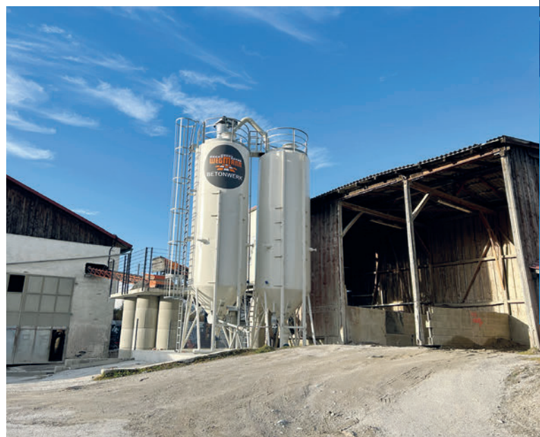
Kniele has also installed two new cement silos.
