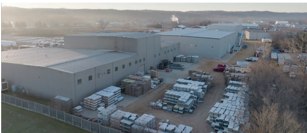
Rochester Concrete Products' new manufacturing plant at their Interlock Concrete location in Jordan MN
